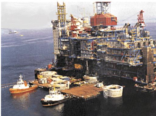
57,000 tons, and provides accommodation for about 200 people and support for drilling equipment weighing about 40,000 tons. When the first model sank in August 1991, the crash caused a seismic event registering 3.0 on the Richter scale, and left nothing but a pile of debris at 220m of depth. The failure involved a total economic loss of about \$700 million.
